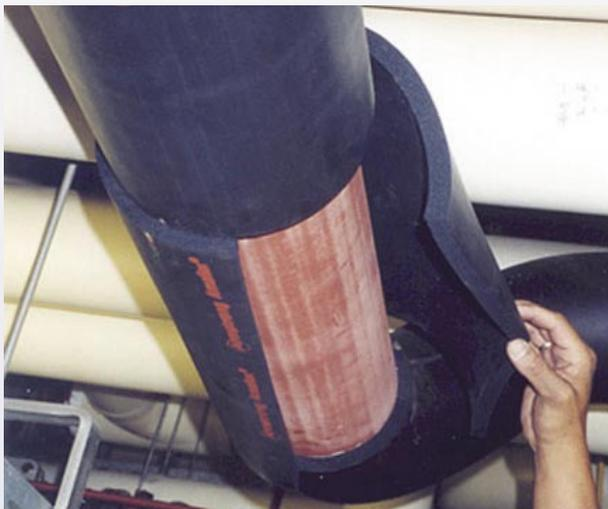
No corrosion even after 25 years. Armaflex installation at Rabo Bank, Amsterdam.
